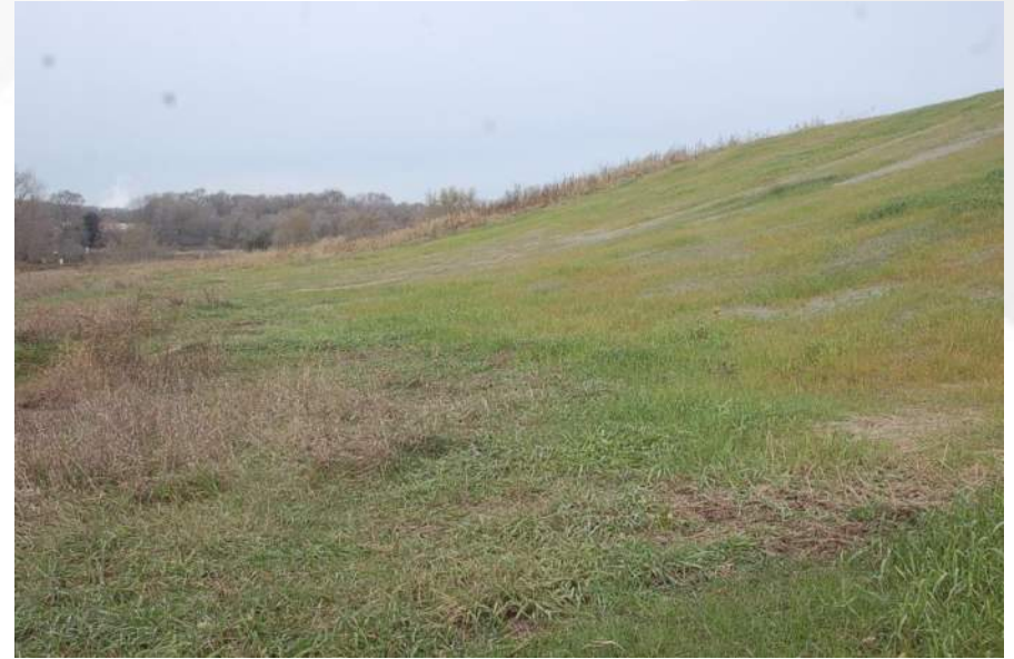
Photo 60 - Cell 2A South Landfill Face
