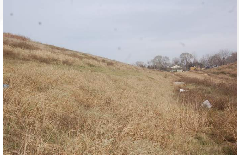
Photo 14 - Cell 3A East Landfill Face
