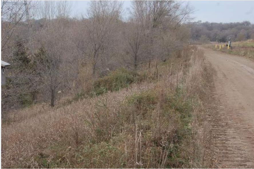
Photo 49 - Cell 2A/2B South Perimeter Berm
