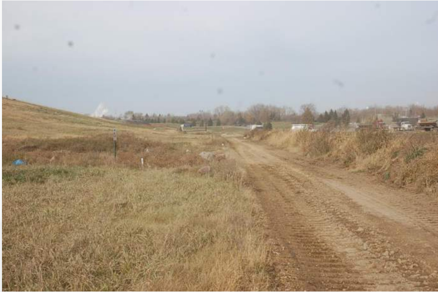
Photo 7 - Cell 3A North Perimeter Rd/LF Toe
