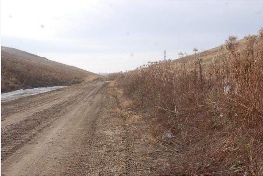
Photo 13 - Cell 3A East Perimeter Rd/LF Toe
