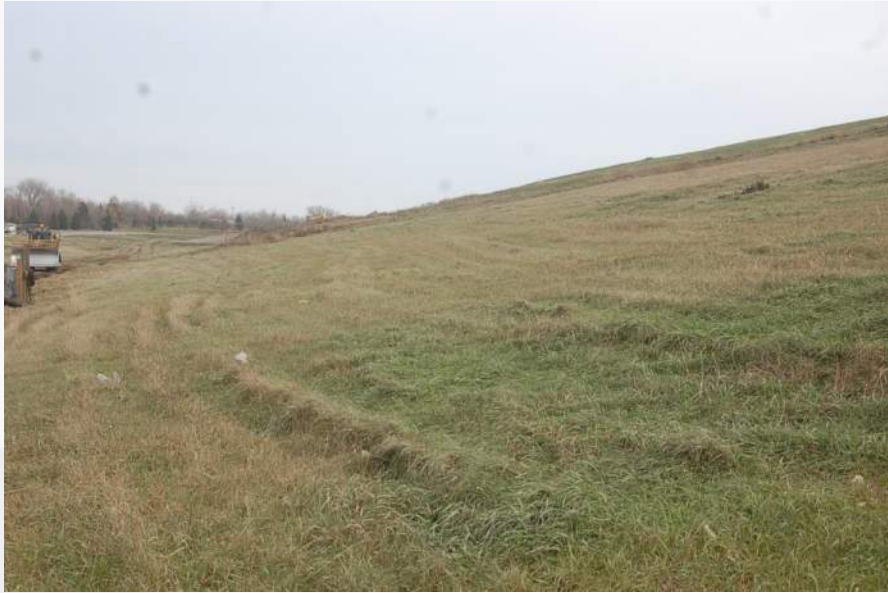
Photo 71 - Cell 1 West Landfill Face
