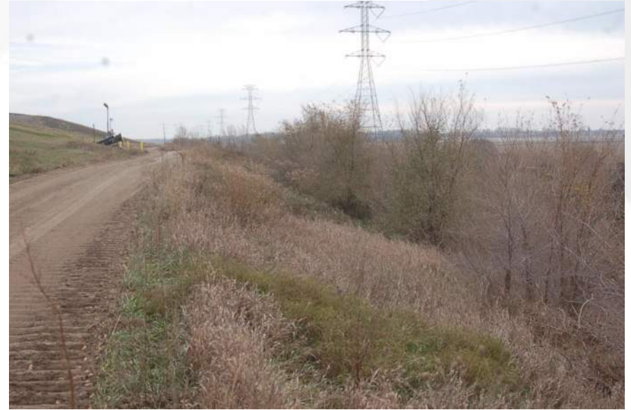
Photo 50 - Cell 2B/2C South Perimeter Berm
