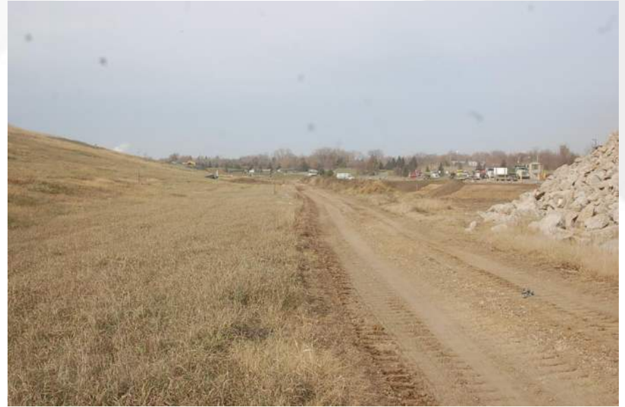
Photo 8 - Cell 3A North Perimeter Rd/LF Toe
