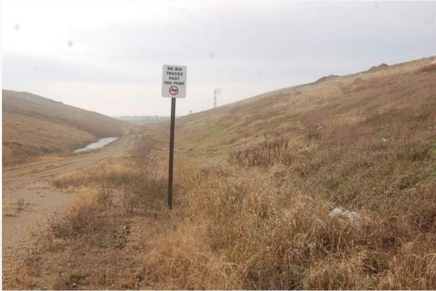
Photo 11 - Cell 3A East Perimeter Rd/LF Toe
