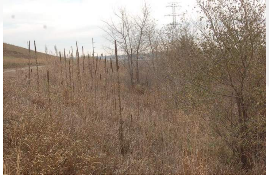
Photo 38 - Cell 2C/2D South Perimeter Berm
