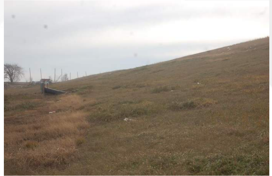
Photo 2 - Cell 3A/3B North Landfill Face
