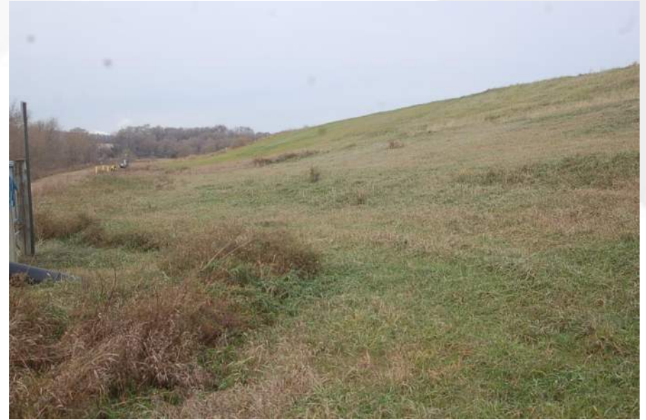
Photo 54 - Cell 2A/2B South Landfill Face
