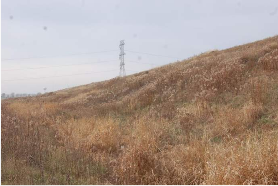
Photo 27 - Cell 3C East Landfill Face
