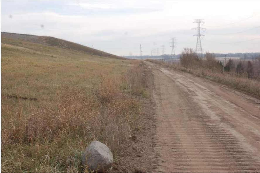
Photo 45 - Cell 2C South Perim Rd/LF Toe
