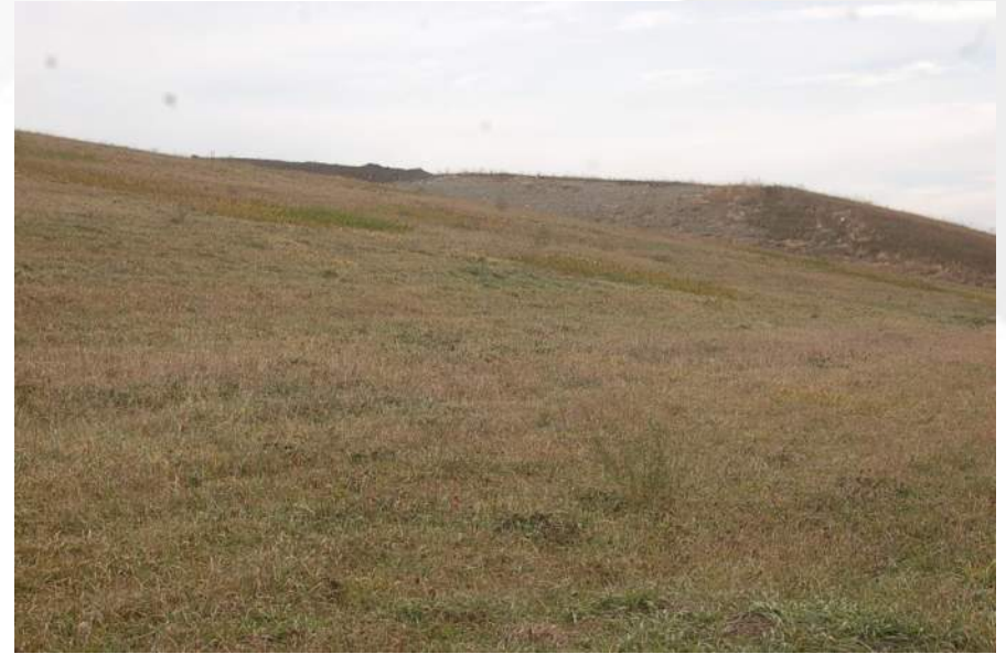
Photo 40 - Cell 2C/2D South Landfill Face
