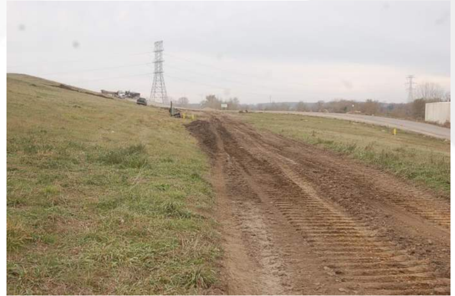
Photo 74 - Cell 1 West Perimeter Rd/LF Toe
