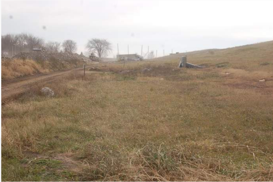
Photo 3 - Cell 3A/3B North Perim Rd/LF Toe
