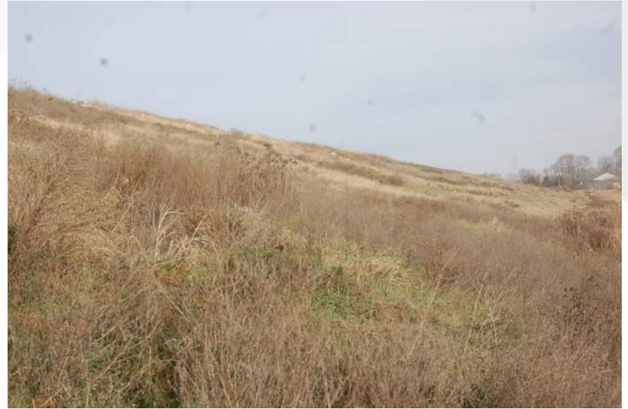
Photo 18 - Cell 3A East Landfill Face
