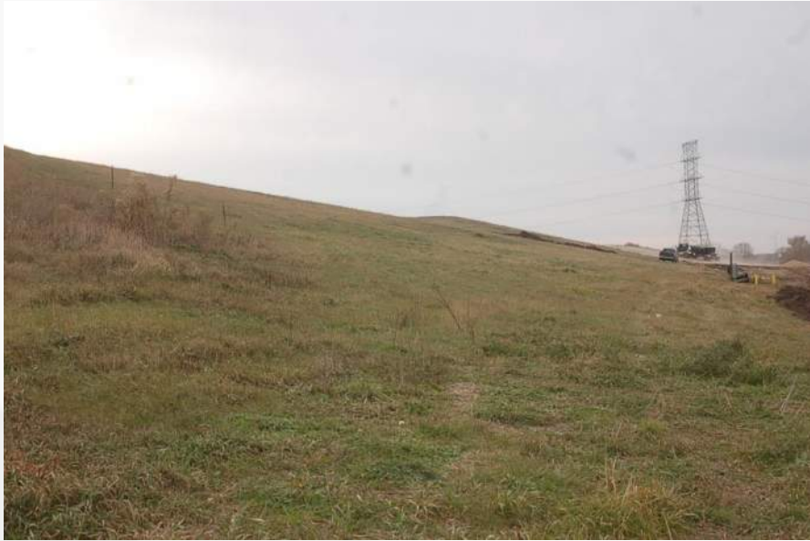
Photo 73 - Cell 1 West Landfill Face
