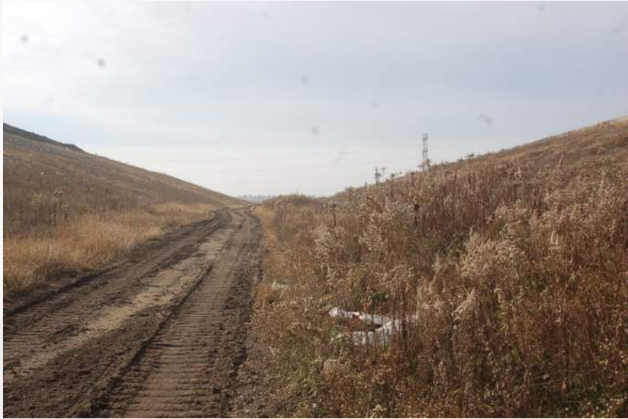
Photo 17 - Cell 3A East Perim RD/LF Toe
