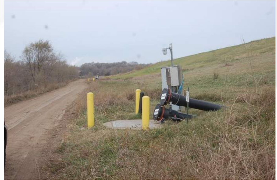
Photo 52 - Cell 2A/2B South Perim Rd/LF Toe
