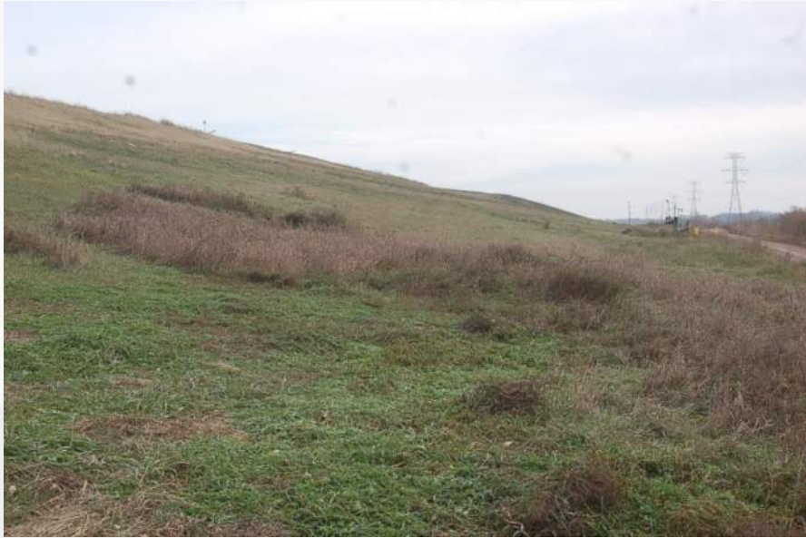
Photo 59 – Cell 2A/2B South Landfill Face
