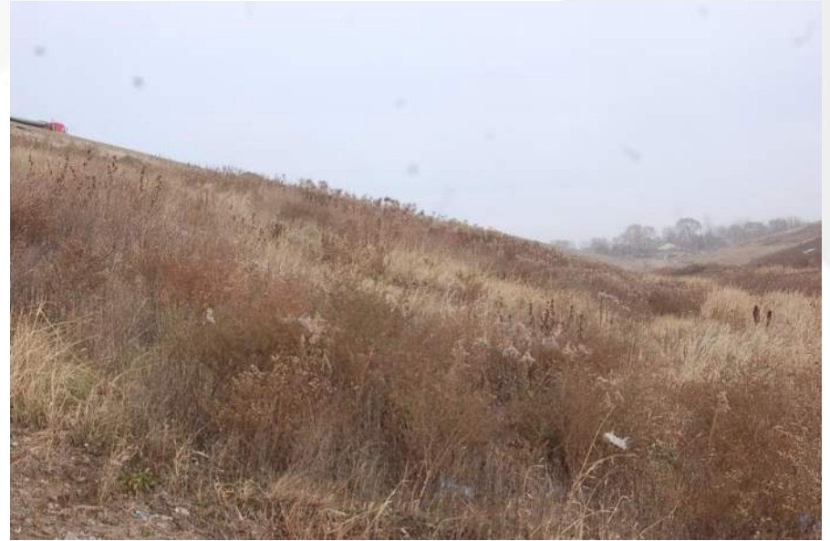
Photo 30 - Cell 3C East Landfill Face
