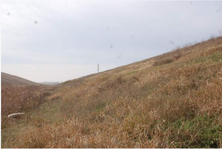
Photo 15 - Cell 3A East Landfill Face
