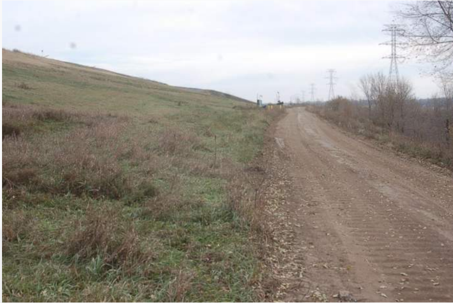
Photo 57 - Cell 2A/2B South Perim Rd/LF Toe
