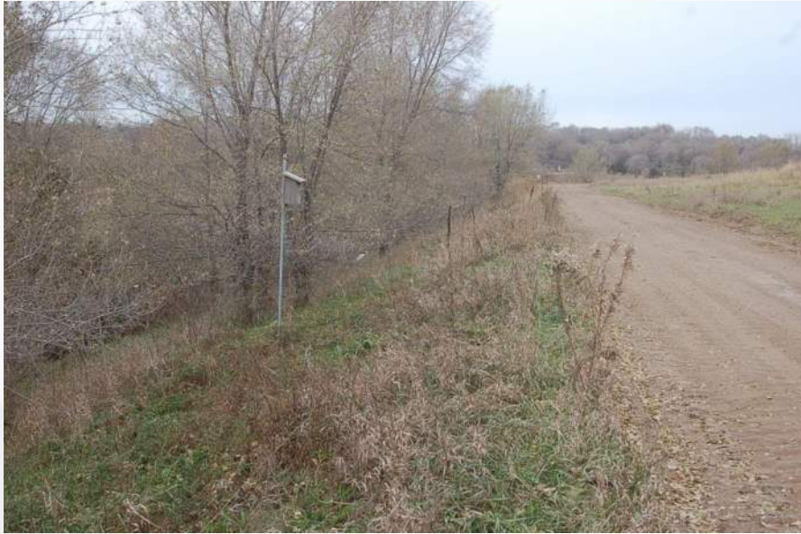
Photo 55 - Cell 2A/2B South Perimeter Berm
