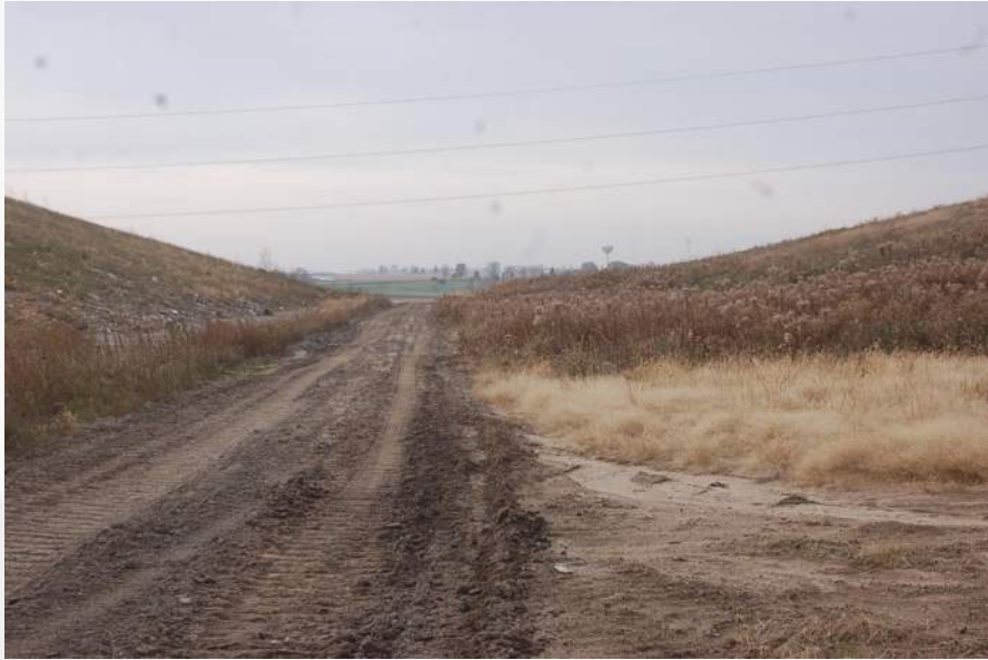
Photo 29 - Cell 2D East Perim Rd/LF Toe
