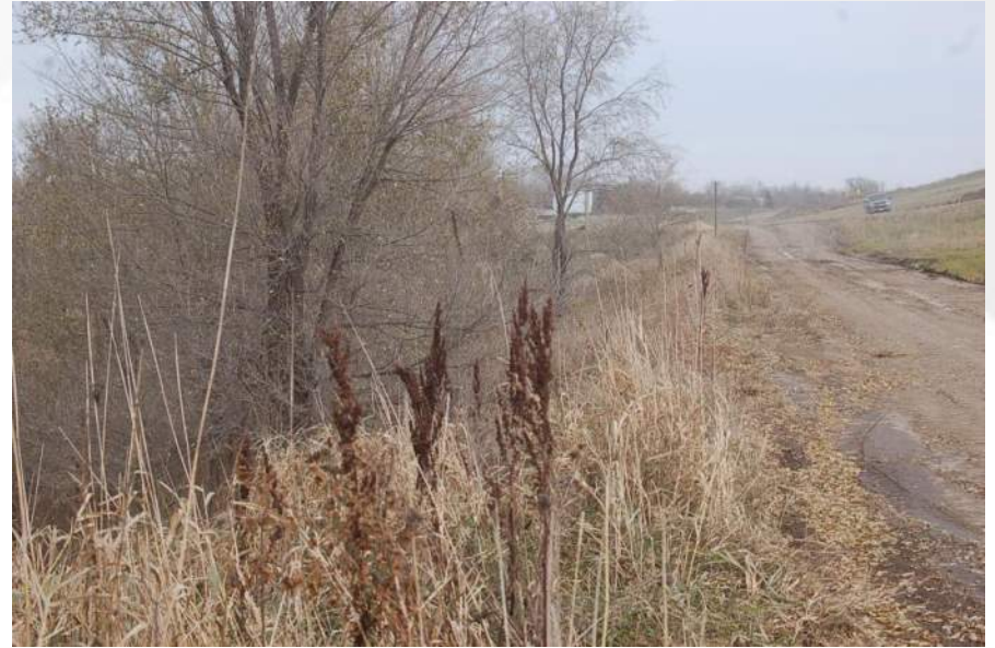
Photo 66 - Cell 2A West Perimeter Berm
