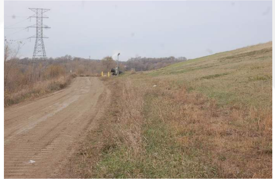
Photo 46 - Cell 2C South Perim Rd/LF Toe
