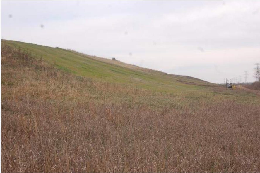
Photo 61 – Cell 2A South Landfill Face
