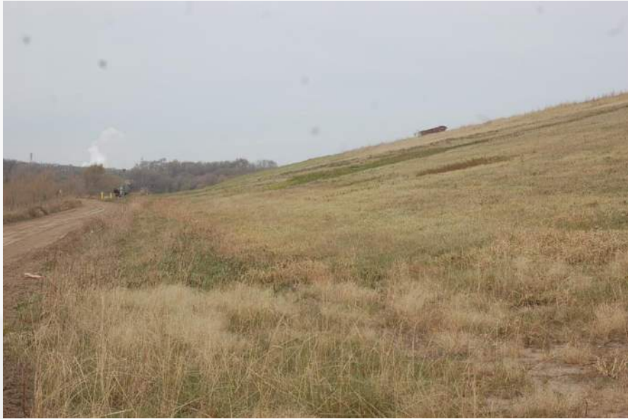
Photo 39 - Cell 2C South Landfill Face
