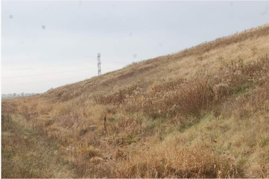
Photo 23 - Cell 3C East Landfill Face
