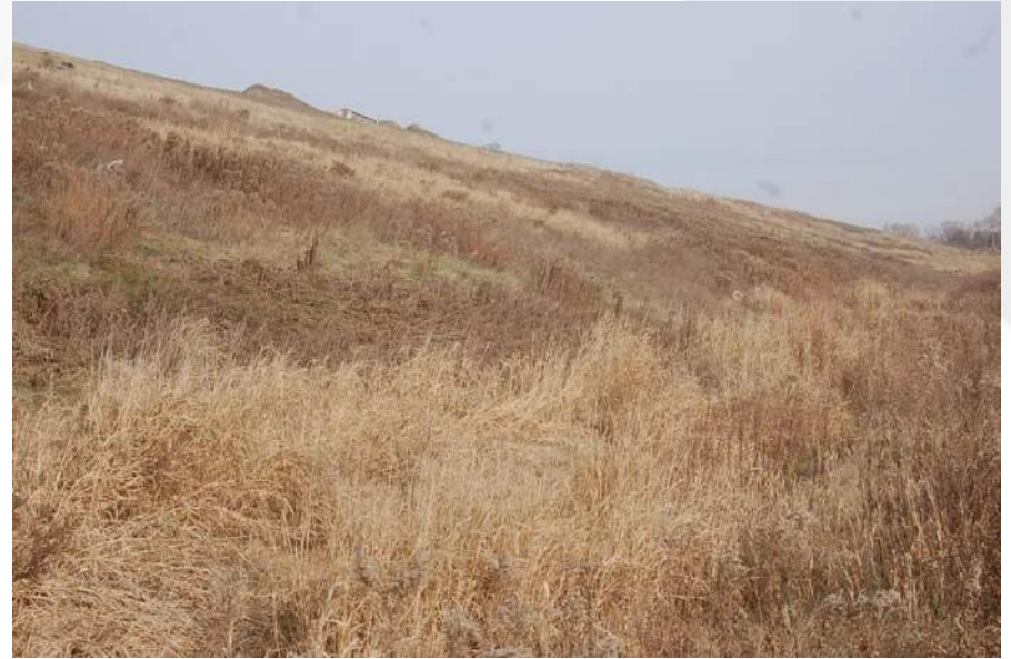
Photo 26 - Cell 3C East Landfill Face
