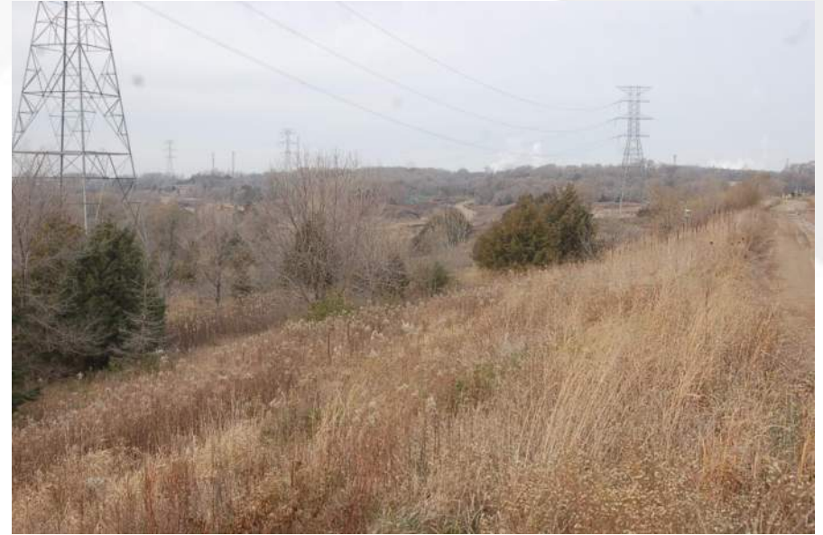
Photo 34 - Cell 2D South Perimeter Berm
