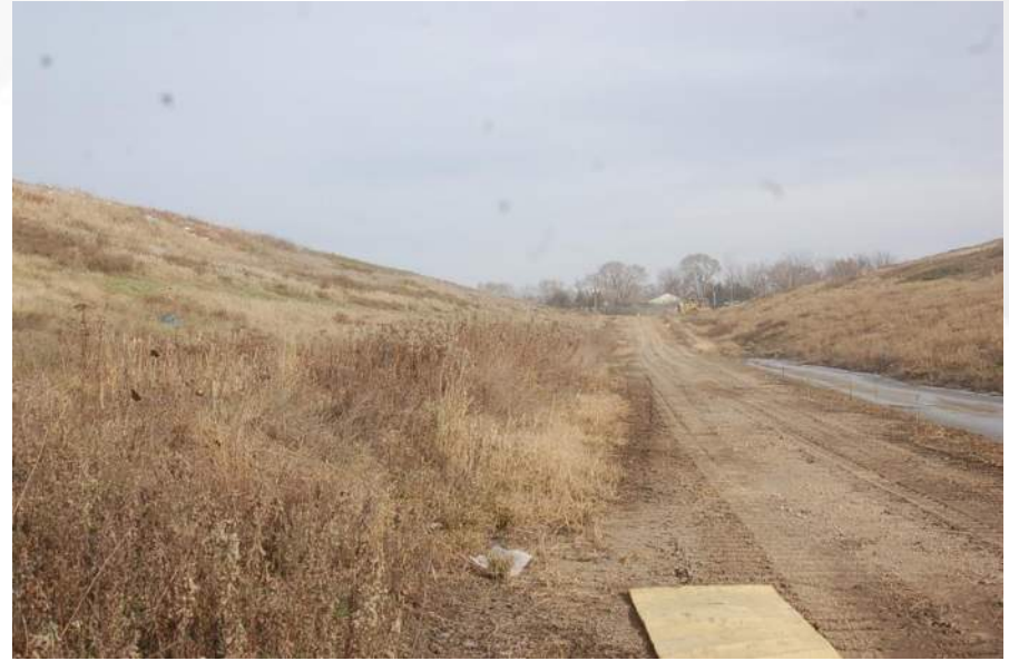
Photo 16 - Cell 3A East Perim RD/LF Toe
