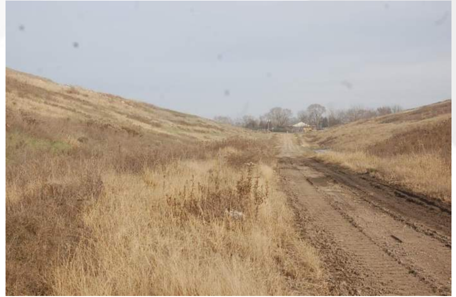
Photo 20 - Cell 3A Perim Rd/LF Toe
