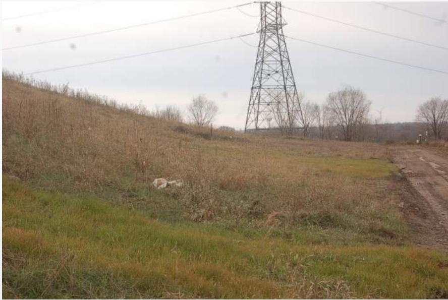
Photo 67- Cell 2A West Landfill Face
