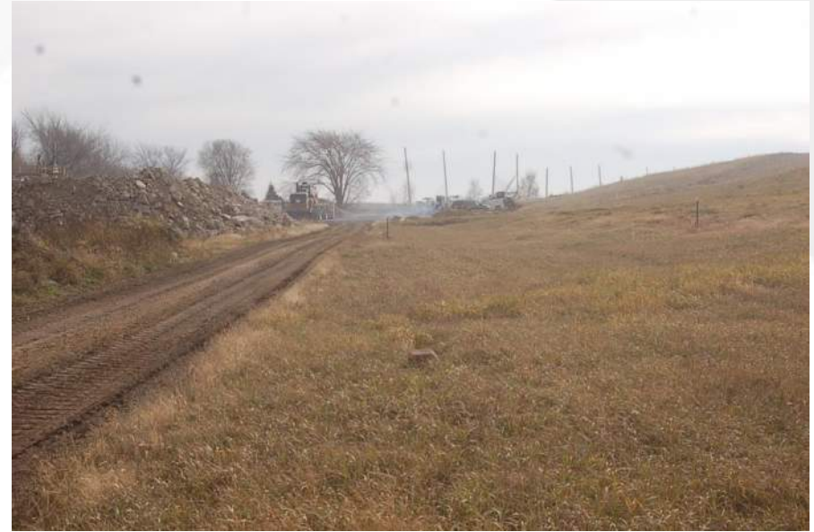
Photo 6- Cell 3A North Perimeter Rd/LF Toe
