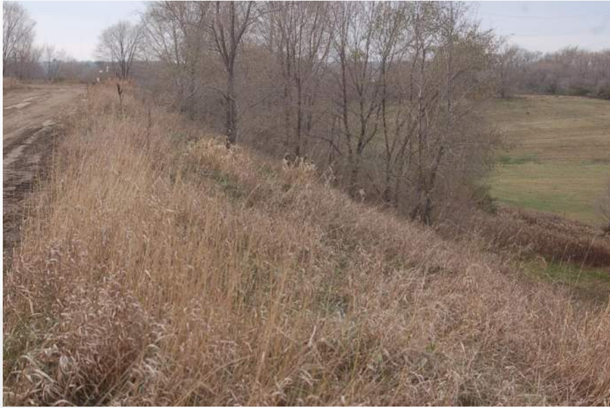
Photo 69 - Cell 2A West Perimeter Berm
