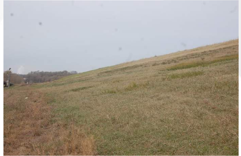
Photo 48 - Cell 2C South Landfill Face
