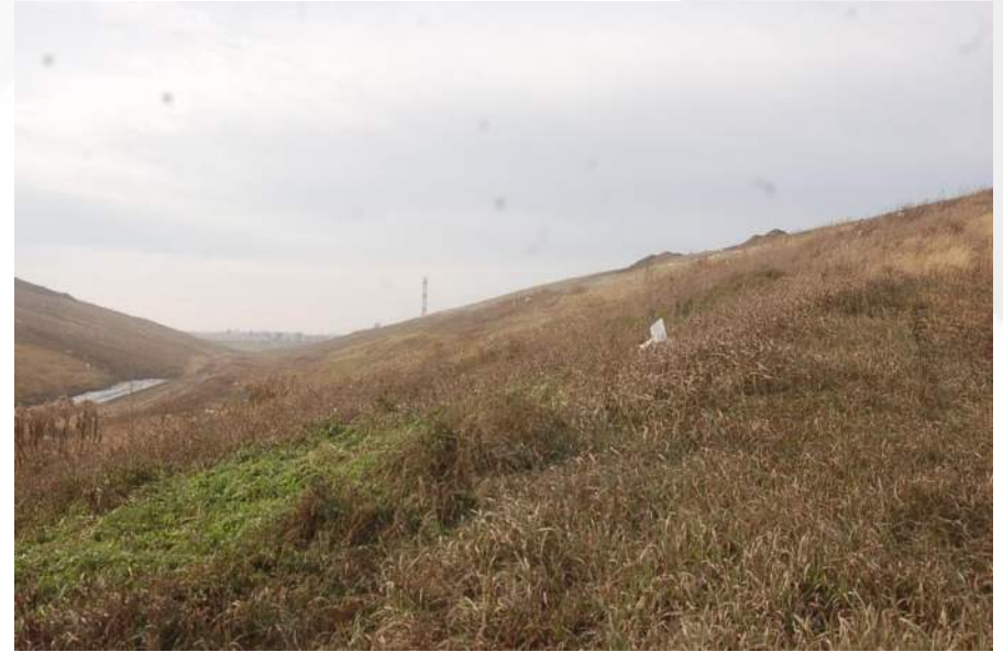
Photo 10 - Cell 3A East Landfill Face
