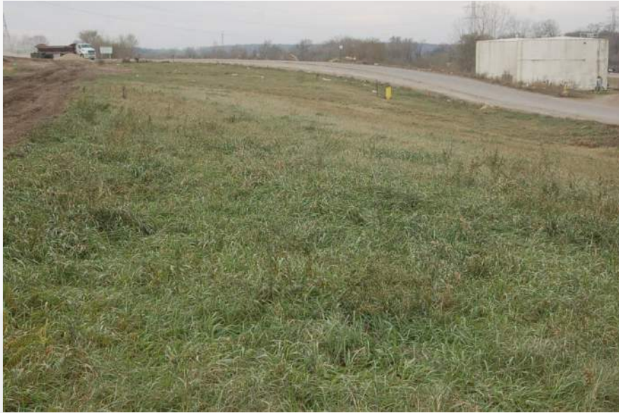
Photo 75 - Cell 1 West Perimeter Berm
