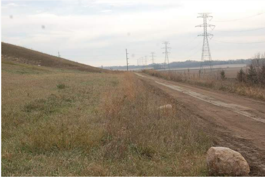
Photo 41 - Cell 2C/2D South Perim Rd/LF Toe
