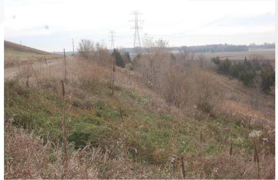
Photo 44 Cell 2C South Perimeter Berm
