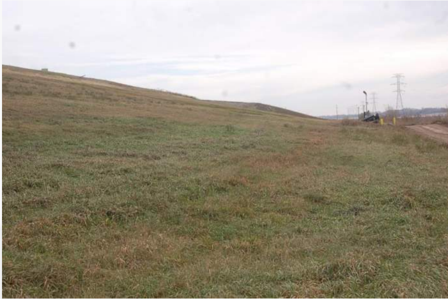
Photo 53 - Cell 2B/2C South Landfill Face
