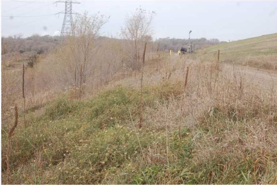
Photo 43 Cell 2C South Perimeter Berm
